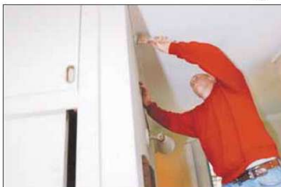
Joe Chetta joins other St. Jerome parishioners as they refurbish a home on Wake Robin Road in Norwalk. The 30 people from St. Jerome made up one of 116 teams who renovated 94 homes and community centers this month.
